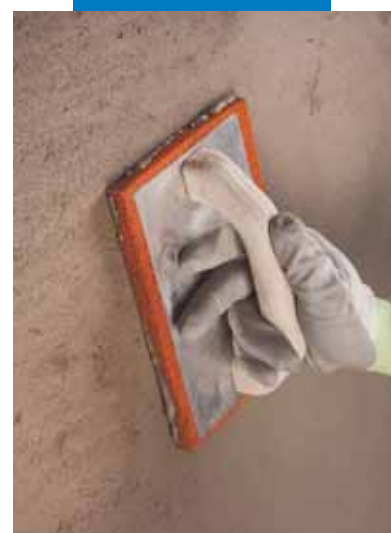
Tamping Planitop Smooth & Repair
