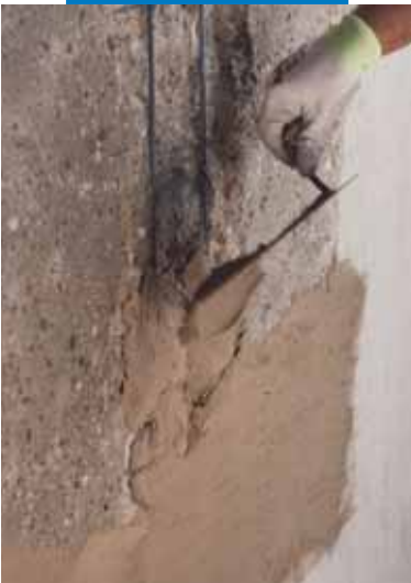
Application of Planitop Smooth & Repair by trowel
