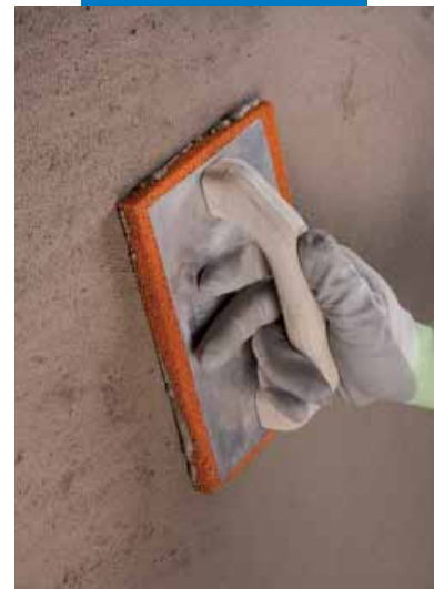
Tamping Planitop Smooth & Repair
