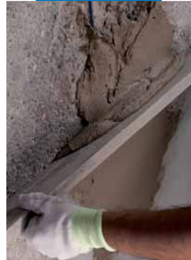
Smoothing of Planitop Smooth & Repair with a straight edge
