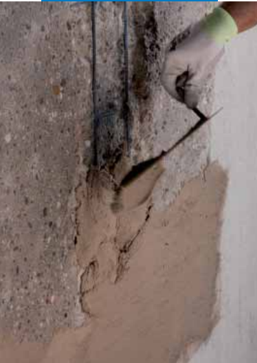
Application of Planitop Smooth & Repair by trowel
