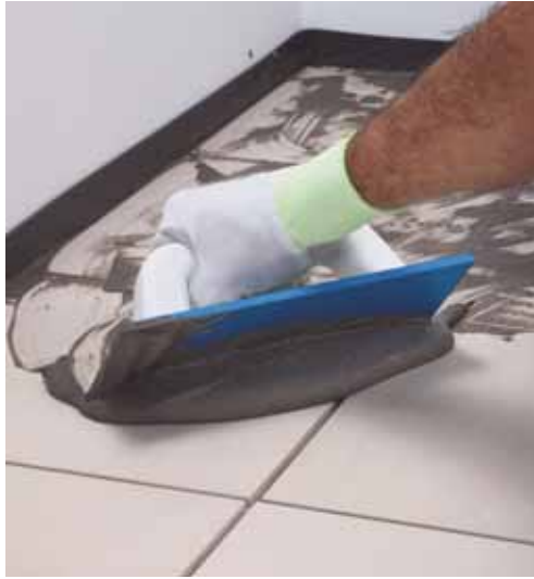
Grout the surface of the room
