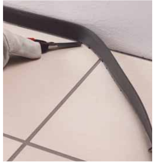
Once the grout has hardened, trim the perimeter of the Mapesonic Strip to remove the excess
