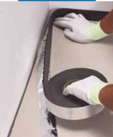
Apply Mapesonic Strip adhesive tape around the perimeter of the room
