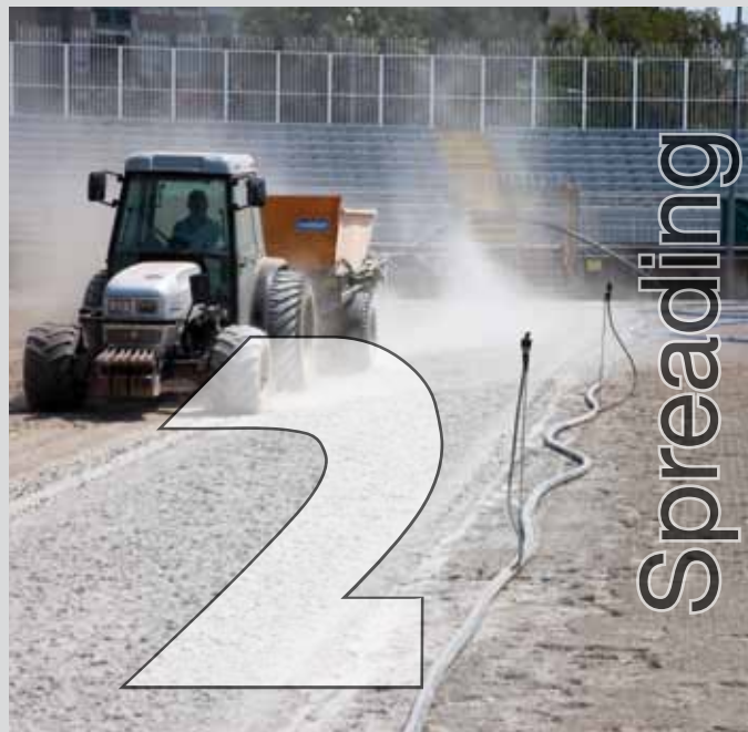
Spreading on the Mapesoil 100 with a sandblaster
