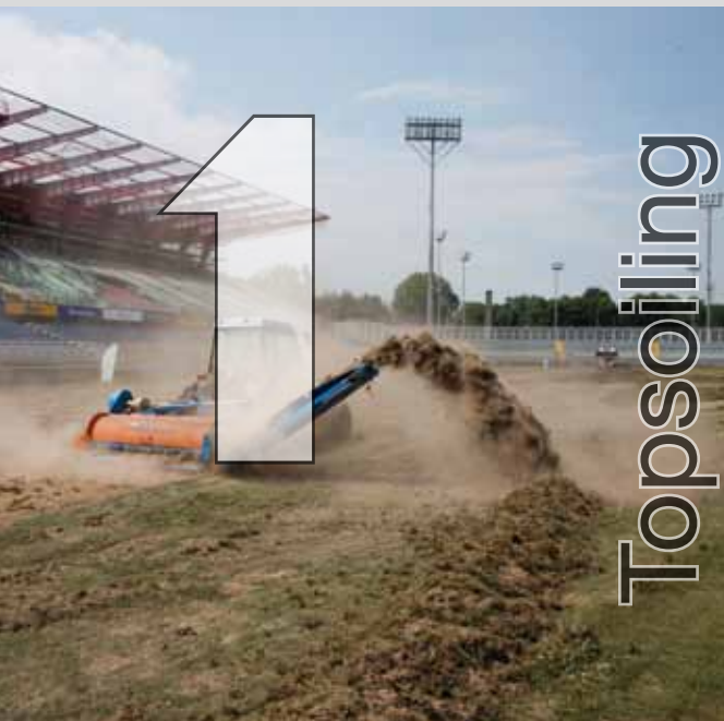
Topsoiling of the old natural grass surface
