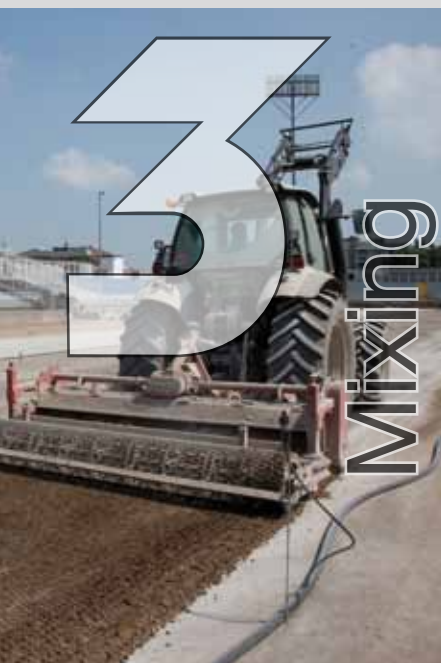
Mixing in the Mapesoil 100 with a plough
