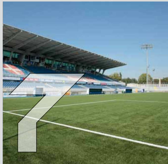
Synthetic grass playing field with horizontal drainage made using Mapesoil 100
