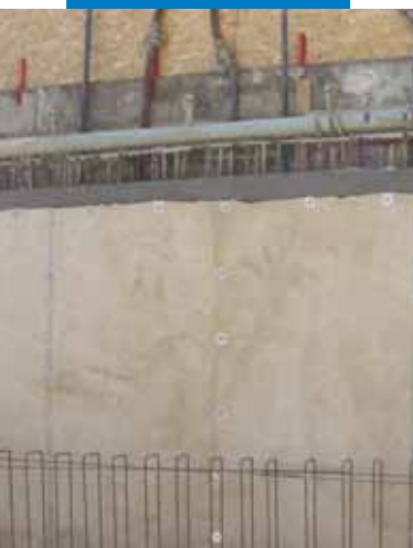
Waterproofing vertical structures against micro-piles
