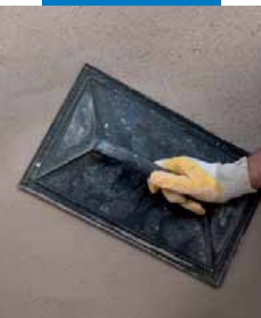
Levelling the render
