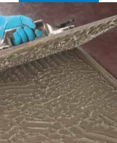
Checking buttering on the back face of tiles
