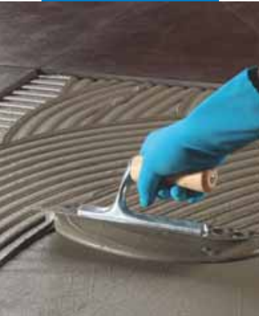
Laying Keraflex Easy on a substrate with a half moon notched trowel with rounded teeth
