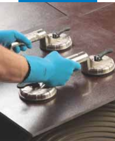
Laying large-sized tiles
