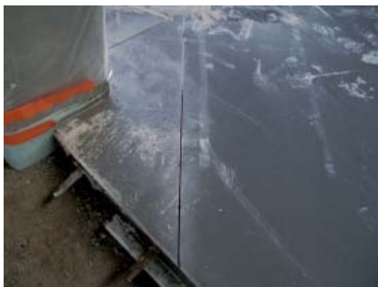
Detail HALFEN Load joint in the column area. NIKE sales center in Laakdal, Belgium.
