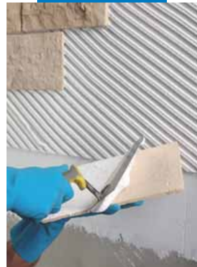
Spreading adhesive on the back of ornamental units
