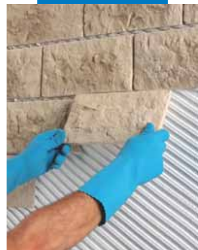
An example of laying ornamental units in lightweight cementitious conglomerate externally
