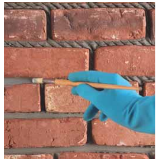
Smoothing the joints with a damp brush
