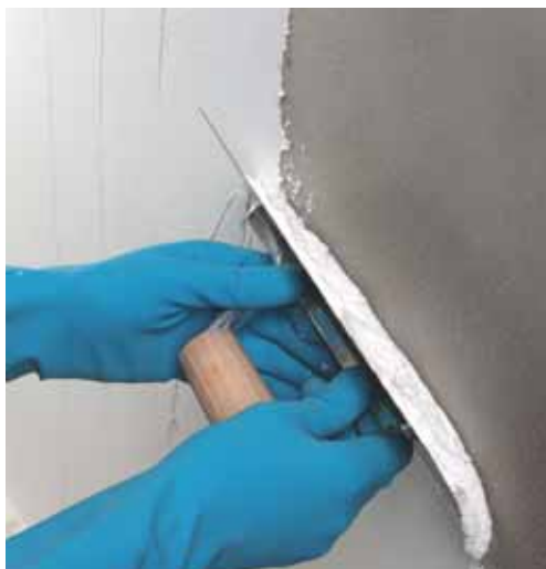
Spreading adhesive to a feather edge on the substrate
