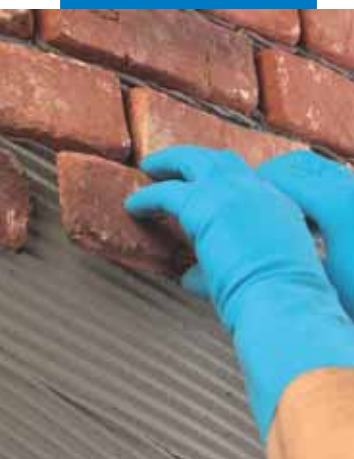
Laying terracotta laths
