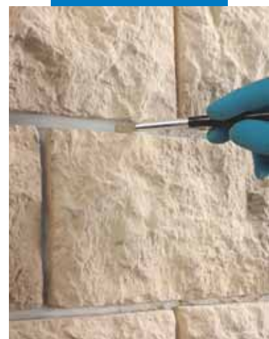
Smoothing the joints with a damp brush
