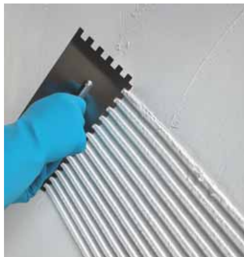
Spreading white Fix & Grout Brick diagonally with a No. 10 notched trowel
