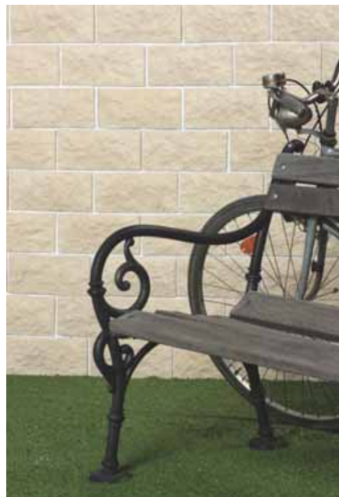
An example of laying ornamental units in lightweight cementitious conglomerate externally
