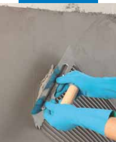
Spreading grey Fix & Grout Brick diagonally with a notched trowel
