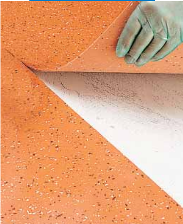
Installation of PVC with Adesilex G20
