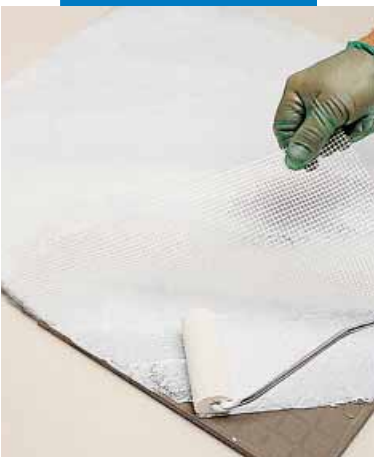
Bonding of reinforcing mesh on the backing of ceramic tiles
